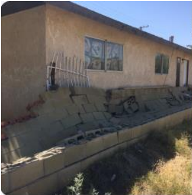
Figure 23. Collapsed cinder block walls of a masonry house (Source: Karen Hua via Twitter)
