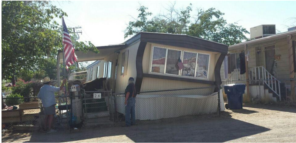
Damaged mobile home in Ridgecrest, CA during the M 6.4 earthquake. Photo by Darla A. Baker / The Californian .
