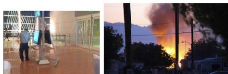
Nonstructural damage at McCarran Airport in Vegas [6]
