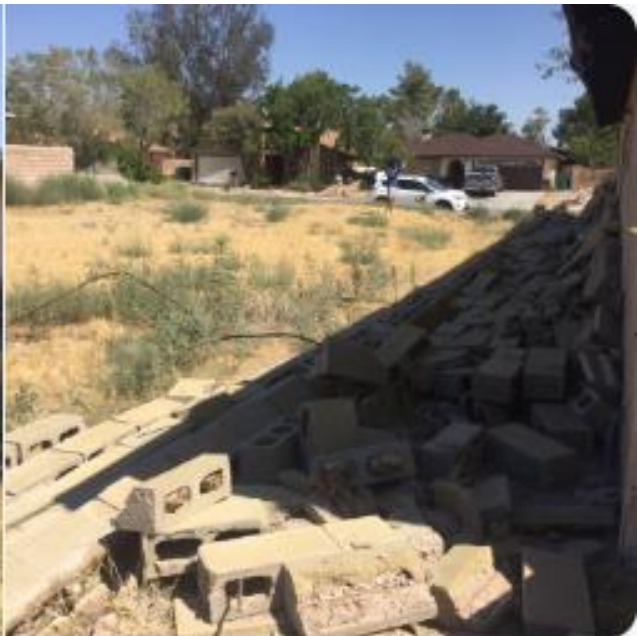
Figure 23. Collapsed cinder block walls of a masonry house (Source: Karen Hua via Twitter)
