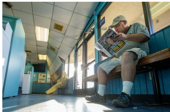
Figure 14. (a) The Daily Independent Newspaper office ceiling damaged during the M 6.4 event (Jessica Watson, AP); (b) Suspended ceiling partial failure at a laundromat in Ridgecrest after the M 6.4 event (Photo by Terry Pierson, The Press-Enterprise/SCNG)
