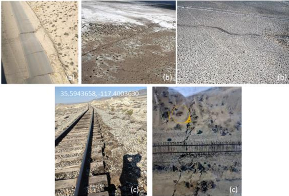
Figure 46. (a) Aerial view of the faulted road on the China Lake NWS base, about 6.5 feet (1.83 m) right lateral (RL) and 3 feet (0.91 m) vertical offset 51 , (b) North-West trending fault rupture measuring 6 feet (1.83 m) of right-lateral offset on the China Lake NWS base 52 , and (c) Bent railroad track due to the fault rupture , close to 3 feet (0.91 m) of RL offset 53
