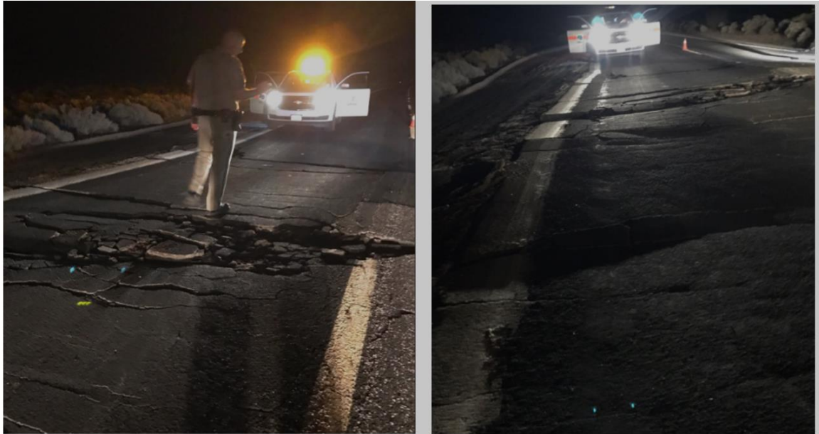
Figure 48. Multiple ground cracks along SR 178 (Source: Caltrans8 Twitter page 56 , taken from the VERT report, Appendix B)
