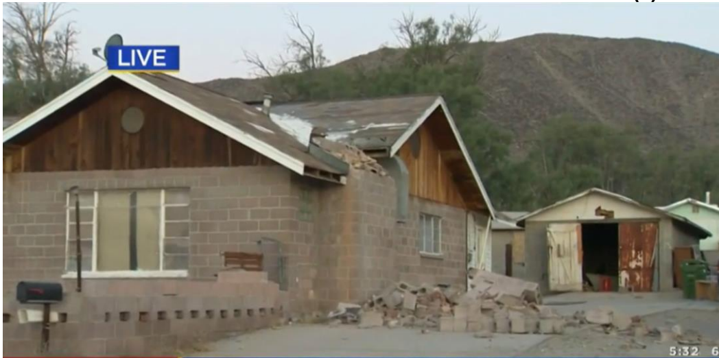
Figure 21. Damage to a masonry houses in Trona after the M 7.1 earthquake (Sources:a) Rob Mcmillan via Twitter, b) CBS Los Angeles)
