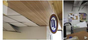
Daily Independent Newspaper office damage [6] Credit: Jessica Weston (AP)
