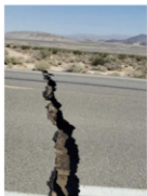
The California Transportation Agency said all repairs have been made and all roads are now open - July 6, 7:30 am [9]
