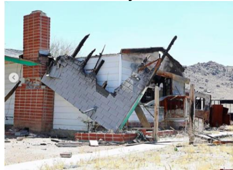
(c) Fire damage after M 7.1 event
